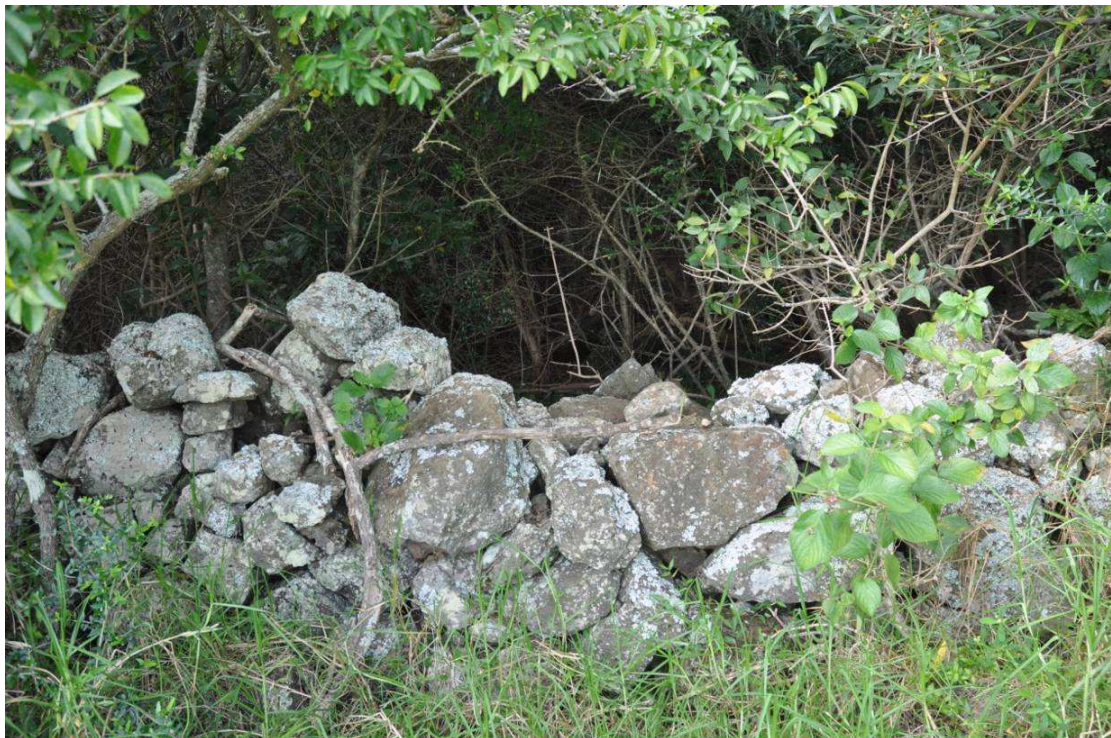
Figure 4.4 Close up of a dry stone wall that lined the boundaries of the study area. (Source: GML 2012)
